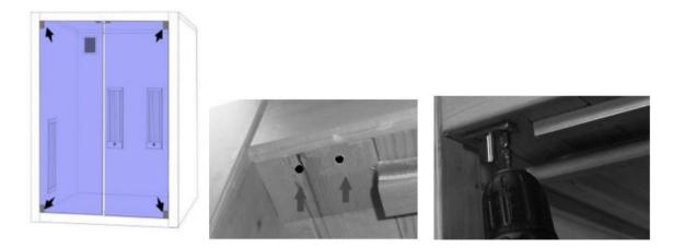
Insert the main part into the base of the hinges and remove the hex screw from the main part, install the door on the hinges, make sure the door holes line up with the hinges, then screw in the hex screws to fix the glass, make sure the hex screws are facing inward.
