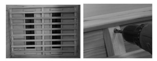
G. installation of glass FRONT PLATE
