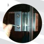
**Note:** The door is heavy. When installing them, it is advisable to support them with a firm, adequately sized pad so that you can seat and tighten the hinges precisely and without much effort.
